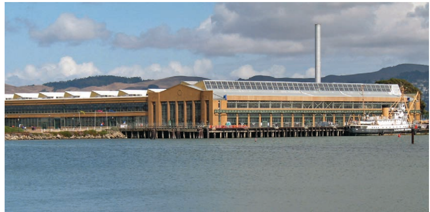
The Kaiser shipyards (top left and right), located on the waterfront west of the Richmond Bay Campus site, were instrumental in the World War II ship building effort. The newly renovated Ford Assembly Building (bottom), was formerly a Ford Motor Company Assembly Plant that during World War II was converted to war-time production use.
