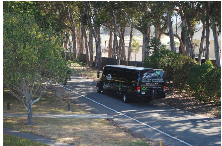
Many of the existing roads lack curbs, gutters and sidewalks.
